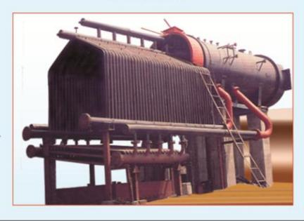
A Typical CTD Model Boiler (Manual Firing cum FBC Firing) Under Erection
